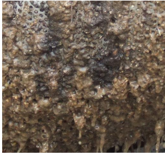
Drain deck above blocked by fat
